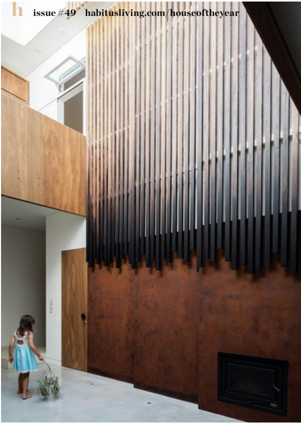
LEFT Timber battens screen the upstairs master bedroom from the atrium.
